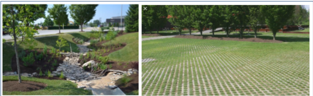
Figure 5-3. Examples of green infrastructure (left: retention basin; right: permeable pavement) that mitigates flooding and high temperatures while allowing infiltration to help replenish the local groundwater system during drought conditions.
