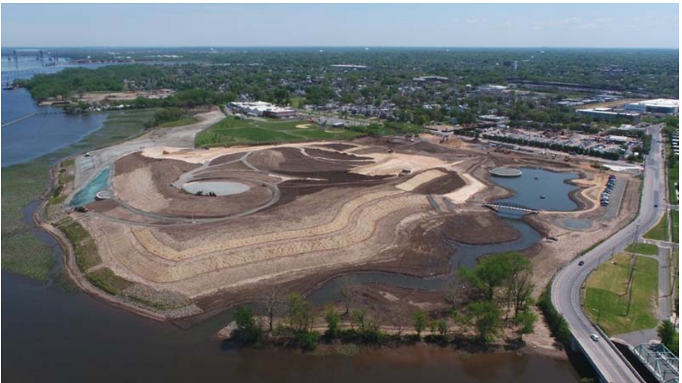
Figure 5-11. Cramer Hill Waterfront Park ongoing development facing east (May 2020).
