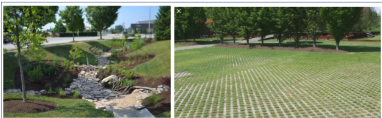
Figure 5-3. Examples of green infrastructure (left: retention basin; right: permeable pavement) that mitigates flooding and high temperatures while allowing infiltration to help replenish the local groundwater system during drought conditions.
