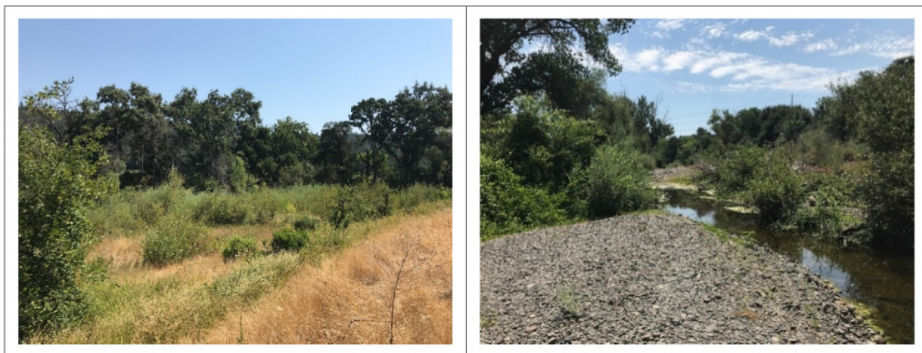
Figure 5-4. Examples of green infrastructure installed to mitigate the effects of and be resilient in the face of flooding (Napa, CA). Flood terrace restoration near the confluence of Sulfur Creek (left) and regraded bank with a wider setback and gravel/cobble bar (right) in St. Helena, CA.
