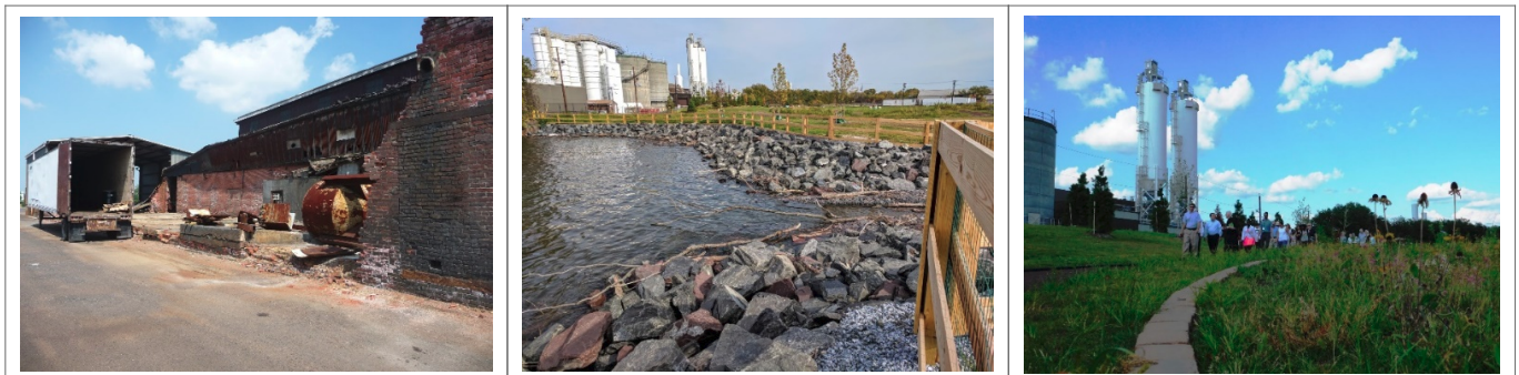
Figure 5-6. The location of Phoenix Park, in Camden, New Jersey, was an abandoned riverside industrial area that has been transformed into a walkable park that provides much needed stormwater management for this dense urban area.
