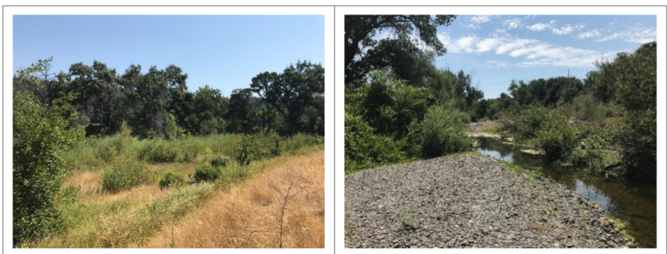
Figure 7-3. Examples of green infrastructure installed to mitigate the effects of and be resilient in the face of flooding (Napa, CA). Flood terrace restoration near the confluence of Sulfur Creek (left) and regraded bank with a wider setback and gravel/cobble bar (right) in St. Helena, CA.
