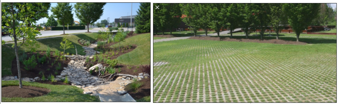
Figure 7-4. Examples of green infrastructure that mitigates flooding (left: retention basin) and high temperatures (right: permeable pavement) while allowing infiltration to help replenish the local groundwater system during drought conditions.
